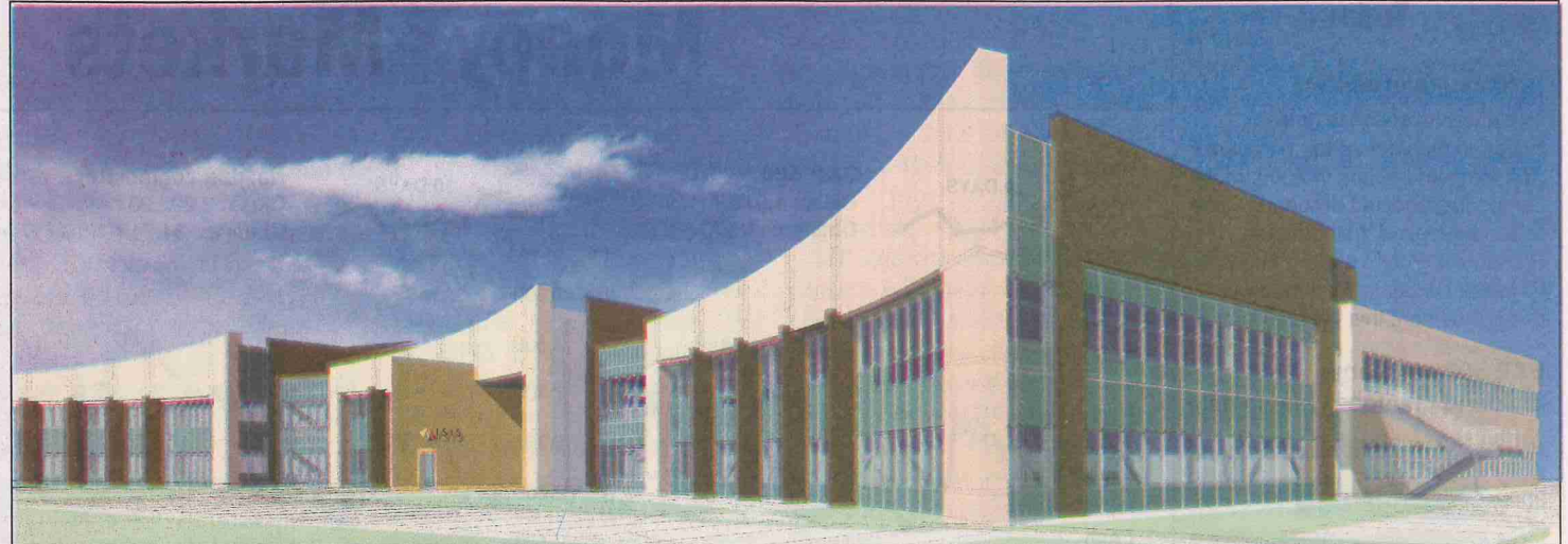
A two-story development of Rancho Bernardo-based BioMed Realty Trust, the new facility will bring BioMed’s total leased space with Isis to approximately 204,700 square feet.
