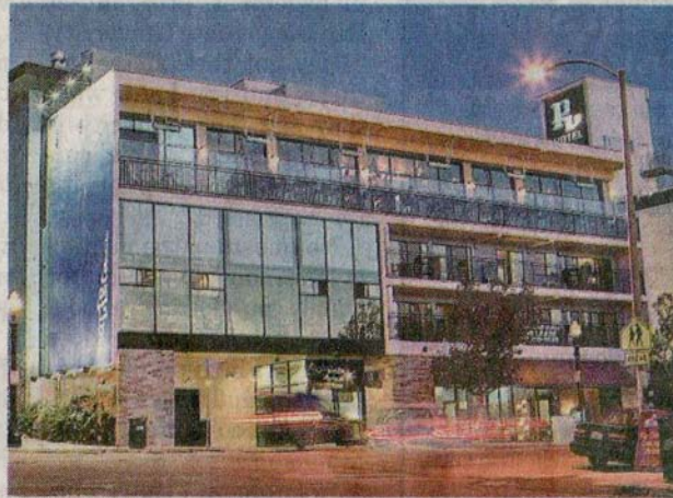
The 189-room Porto Vista Hotel in San Diego's Little Italy neighborhood has a rooftop deck that can be used for a party of 300 guests. PORTO VISTA HOTEL
